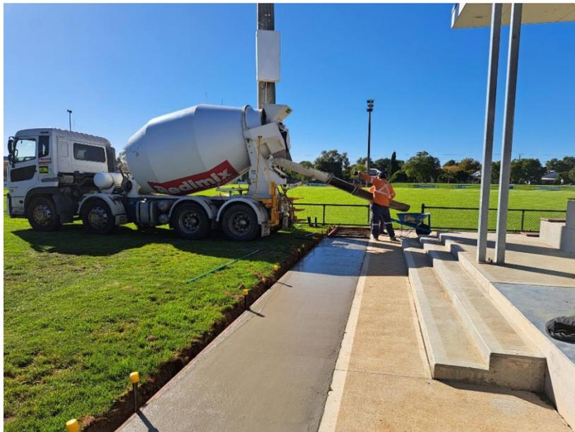
Figure 3: New footpath around the Cale Oval Grandstand
