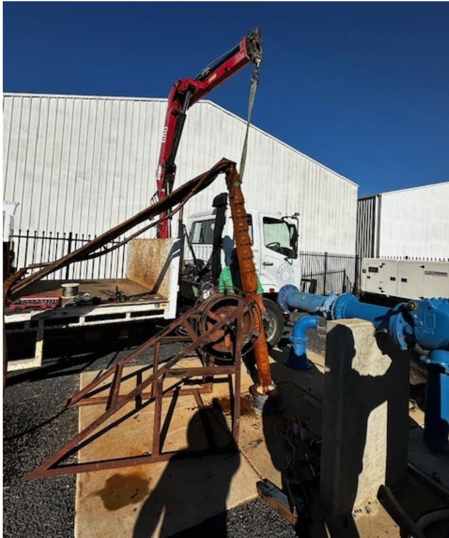
*Figure 1: Narromine Bore 9 was lifted in April. Significant Iron is present on the stainless steel column and pump*
