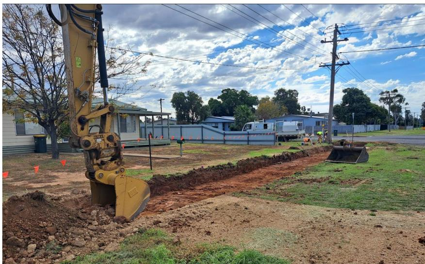
*Figure 7: Installation of kerb and gutter has started on A'Beckett Street.*
