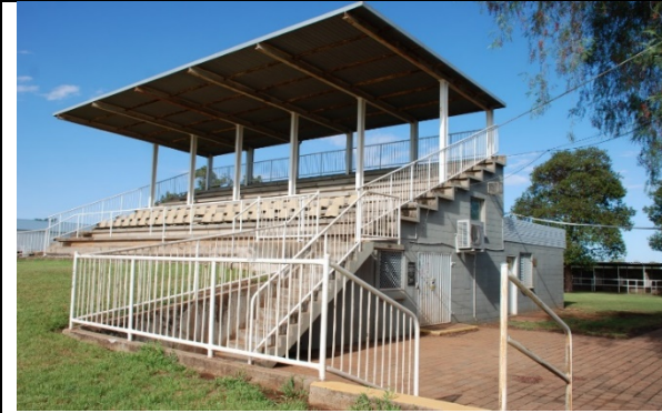
Plate 17: Painted brick grandstand
