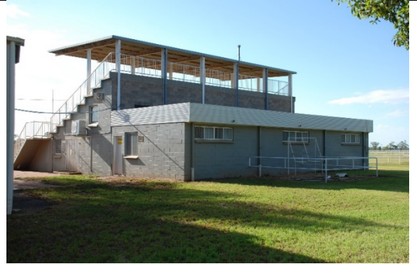
Plate 20: Rear of brick grandstand
