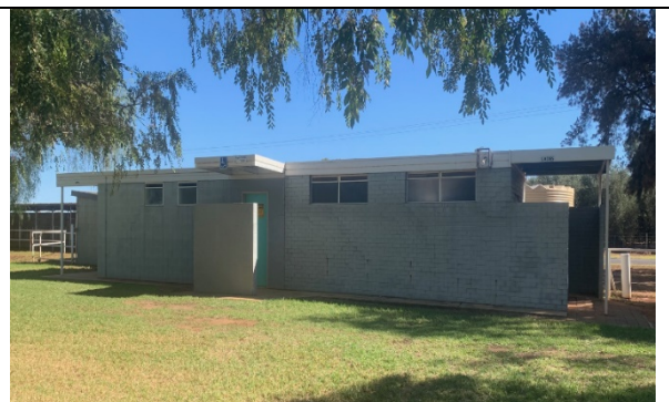
Plate 4: Brick toilet block
